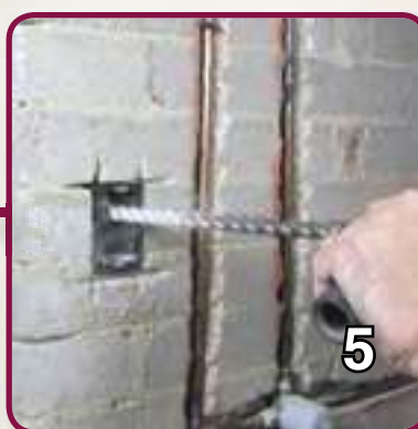
5. Drill hole for cable.
