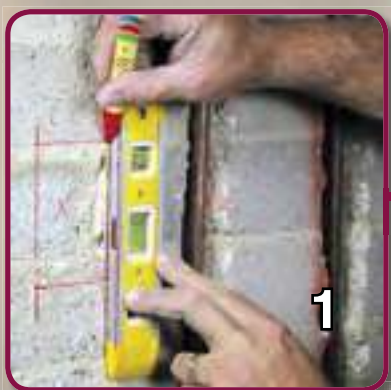
1. Mark out and drill wallbox position.
