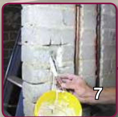
7. Remove wallbox and apply wall/wallbox adhesive.
