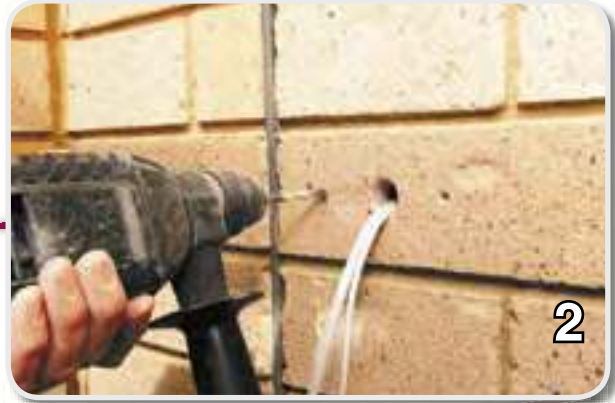
2. Drill out mounting holes.
