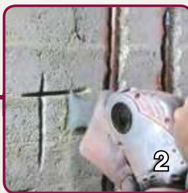
2. Cut or drill out along wall markings.
