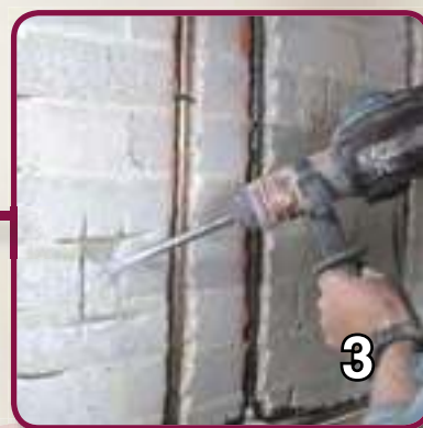
3. Chisel/hammer out brickwork to create wallbox cavity.
