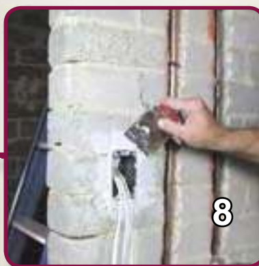
8. Finally, reinsert wallbox and apply wall filler
