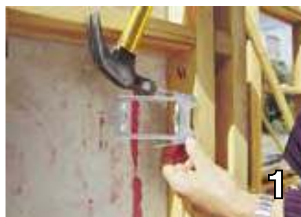
Installation of 155NAR Nail Bracket
