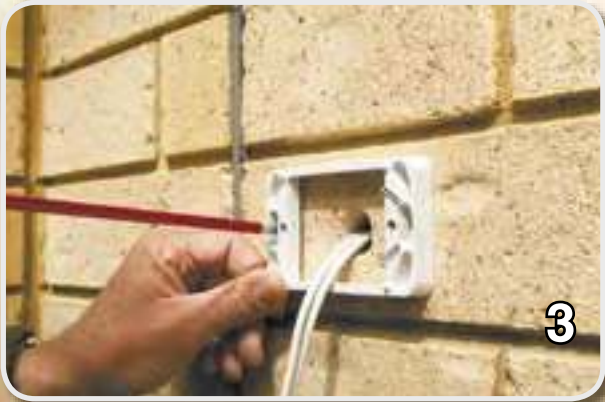
3. Screw fix 2449ASD Spacer Block.
