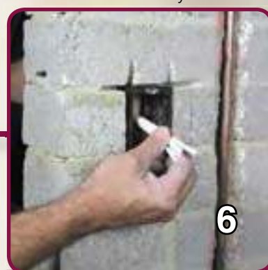
6. Run cable and insert through wall box.
