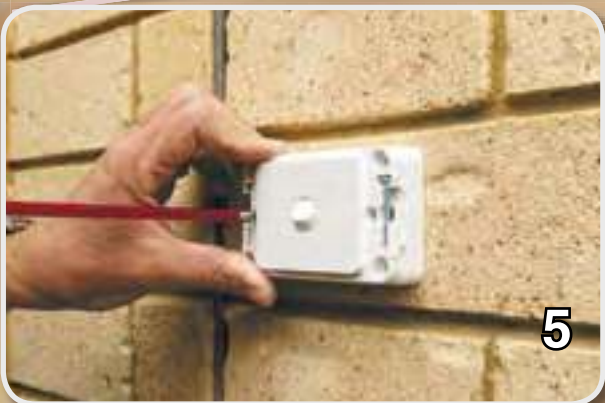
5. Screw fix product to 2449ASD Spacer Block.
